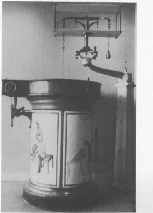
Figs. 1,2: Talabot's thermobalances at Lyon for quality control of Chinese silk
